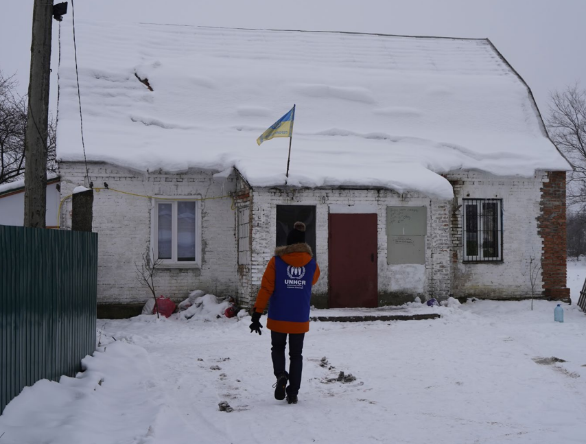
A home in Kyivska oblast that was repaired by UNHCR following shelling at the beginning of the full-scale invasion. © UNHCR/Alina Kovalenko
